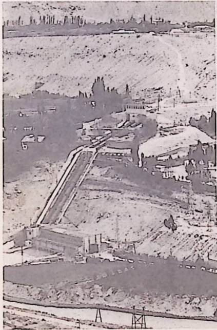
Pamirs region has several large power plants now, and this one on River Gunt is first of many that will utilize mountain streams. But extremely severe winter conditions make construction and maintenance difficult.
