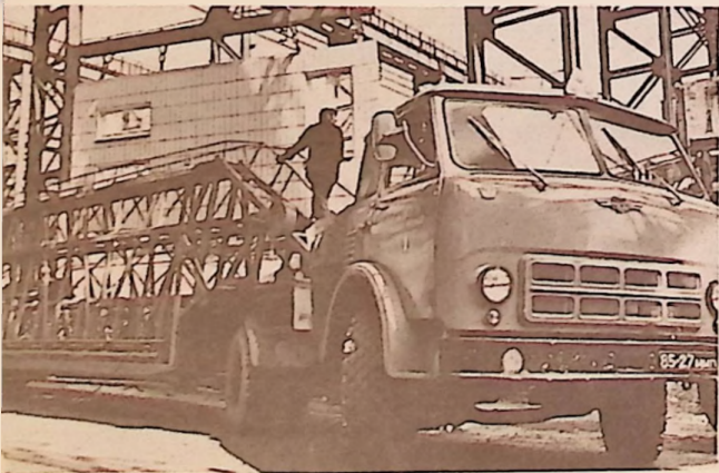
Soviet builders pioneered in "factory-made" housing ... not little one-family homes but full size high-rises. Here they're loading exterior panel on carrier. In USSR you see endless lines of trucks transporting apartments.
