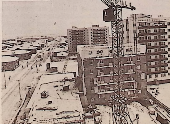
High in Arctic, city of Mimya had to be built on "permafrost". First time anywhere, nine story buildings are going up on piles. Architects in USSR must cope with every climate extreme in designing new housing.
