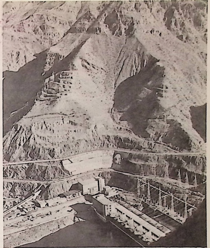
Unique Nurek Power Station literally cut right out of the mountains, using tremendous flow-and-height of Nurek River. Tamed river now irrigates great expanses of farm lands. But it will also be used in other plants.
