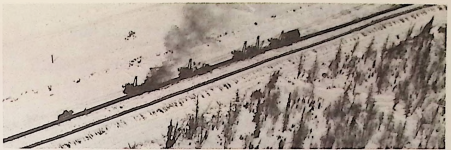
Surprise! Here's that sensational USSR-Europe Gas Pipeline, right where it starts at the enormous Urengoi Deposit. Despite severe Arctic conditions, Soviet workers will finish it ahead of schedule.
